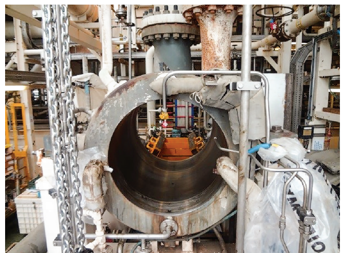
FIG. 9. A compressor casing ready for a new cartridge.
